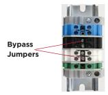
7 Turn on the circuit breaker feeding the Terminal Block. Verify that the circuit breaker does not trip. If a breaker trips, do not proceed with installation until the problem has been resolved. Turn off the circuit breaker again before proceeding with the installation and wiring.
